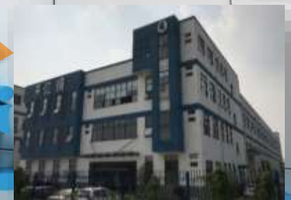
Amould (Automation) SuZhou, China
